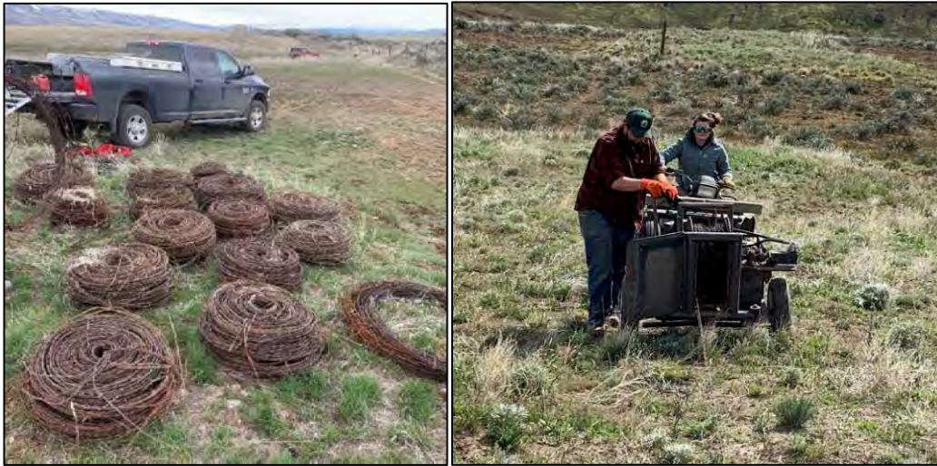
Wire rolled from Mellergaard using mechanical roller. Wire will be staged here and removed in one large load once it has all been rolled. Manager Hughes and Technician Rodriguez rolling wire
