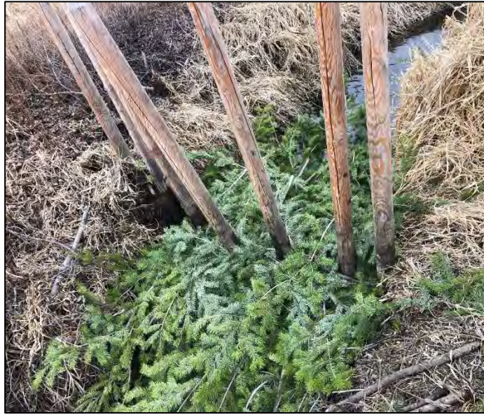
Newly woven BDAs, with limbs pointing both upstream and downstream – Photo by Dupont
