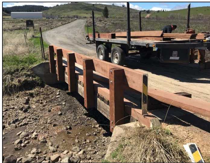
New rails on bridge across Kittitas Reclamation District canal in Joe Watt Canyon
